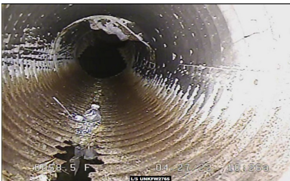
Bottom of the pipe missing (lower section)
