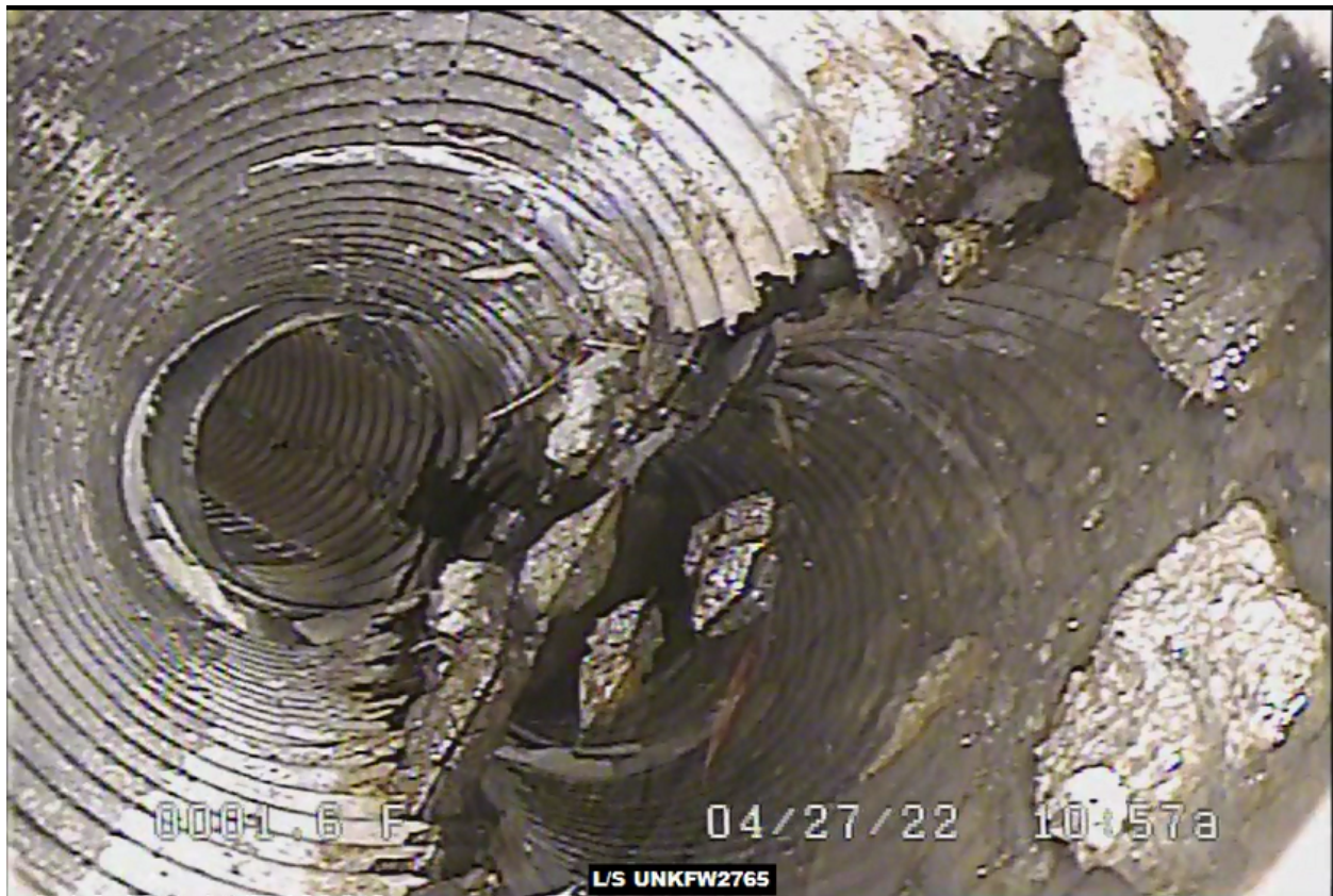
Bottom of the pipe missing (lower section)
