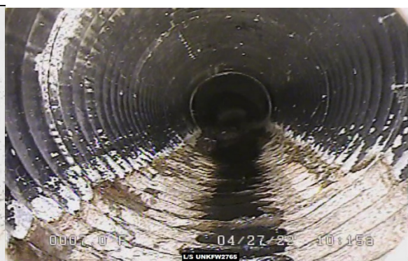
Bottom of the pipe missing (lower section)
